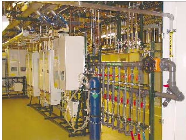
Safety is the primary focus for all gas handling facilities at the PMTC, which included the use of torque elimination fittings in process gas lines.
